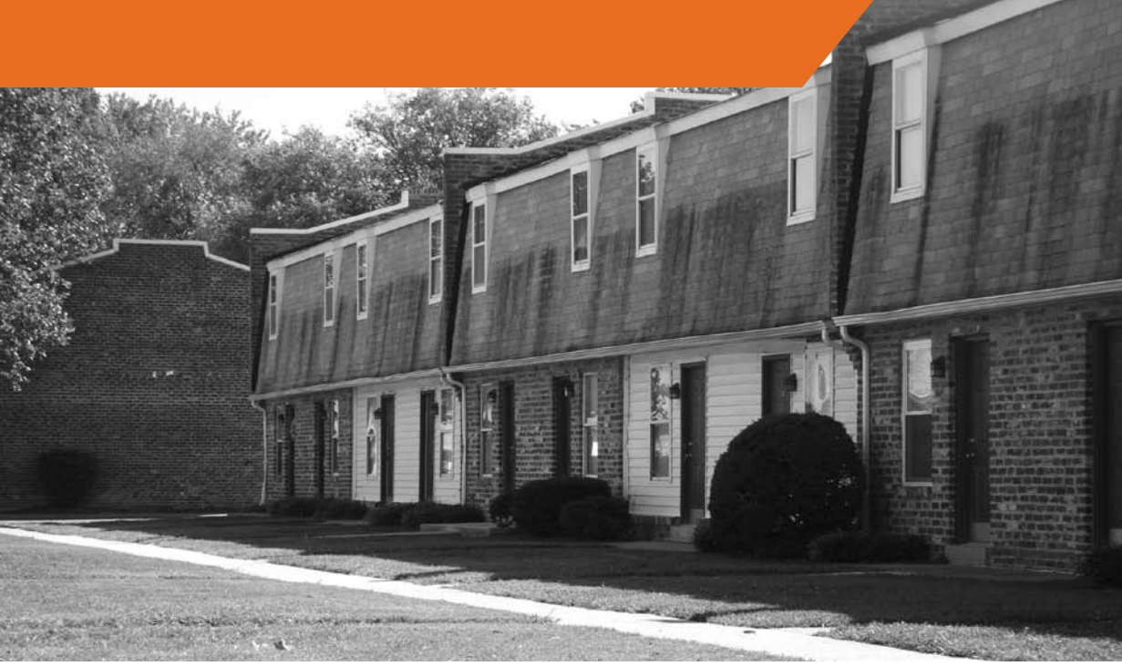
A Lincoln Manor apartment building prior to renovation.
